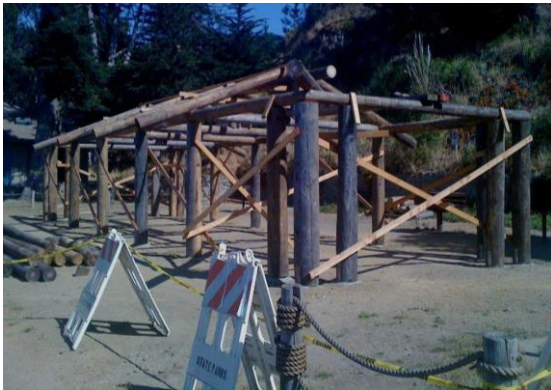
The new Ramada rises near the Visitor Center.
